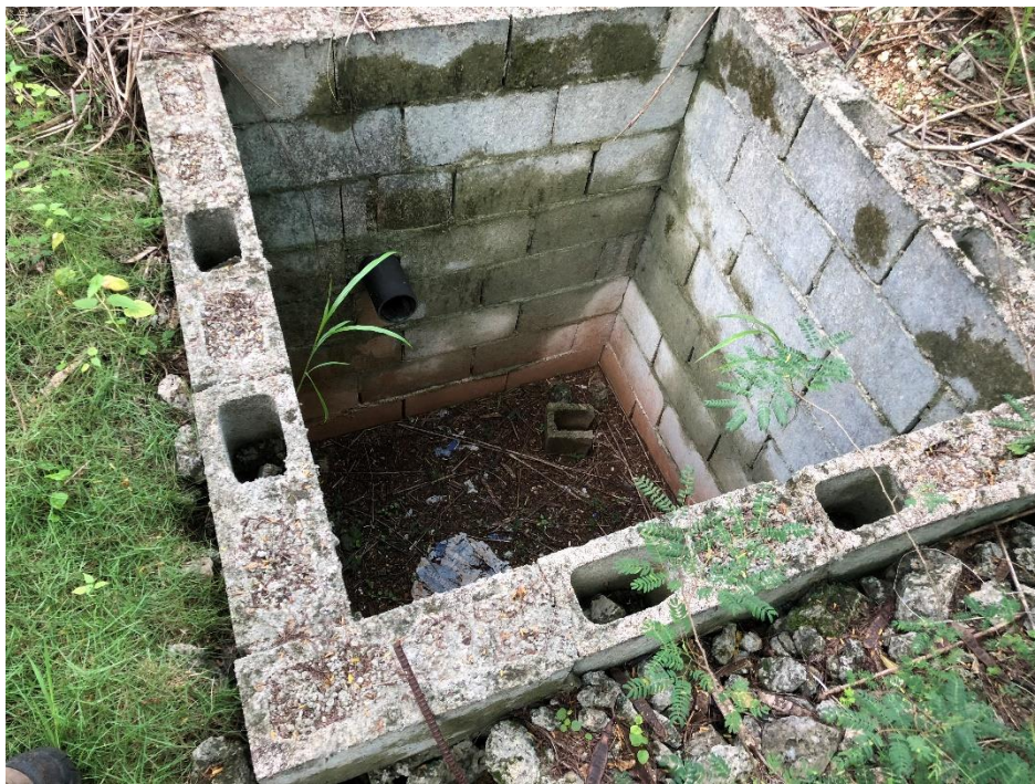
Photo18: Septic tank behind the GPA field office near the southwest boundary of the subject site, Oka Point, Tamuning Guam
