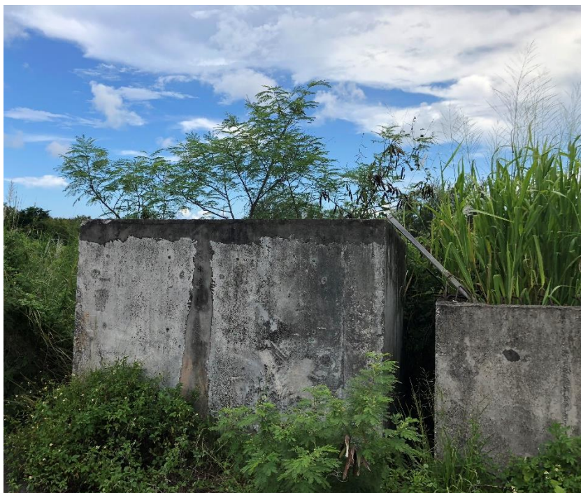
Photo 29: Precast manholes near the southern portion of the subject site, Oka Point, Tamuning Guam
