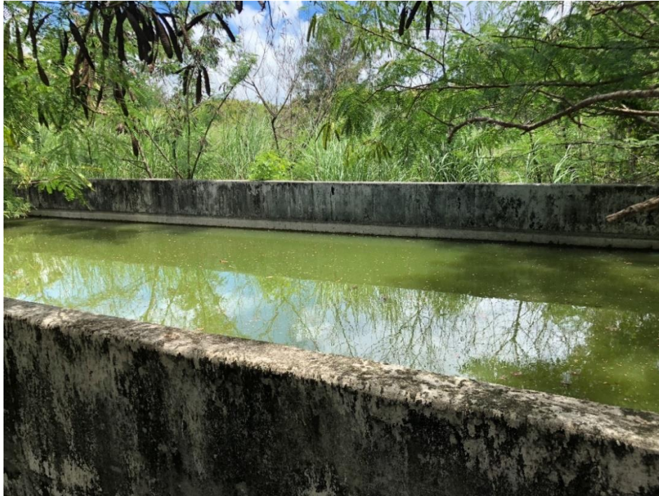
Photo 7: Concrete foundation found near the abandoned generator building that was possibly used as a containment for an Above-ground Storage Tank (AST) at the northwest portion of the subject site, Oka Point, Tamuning Guam
