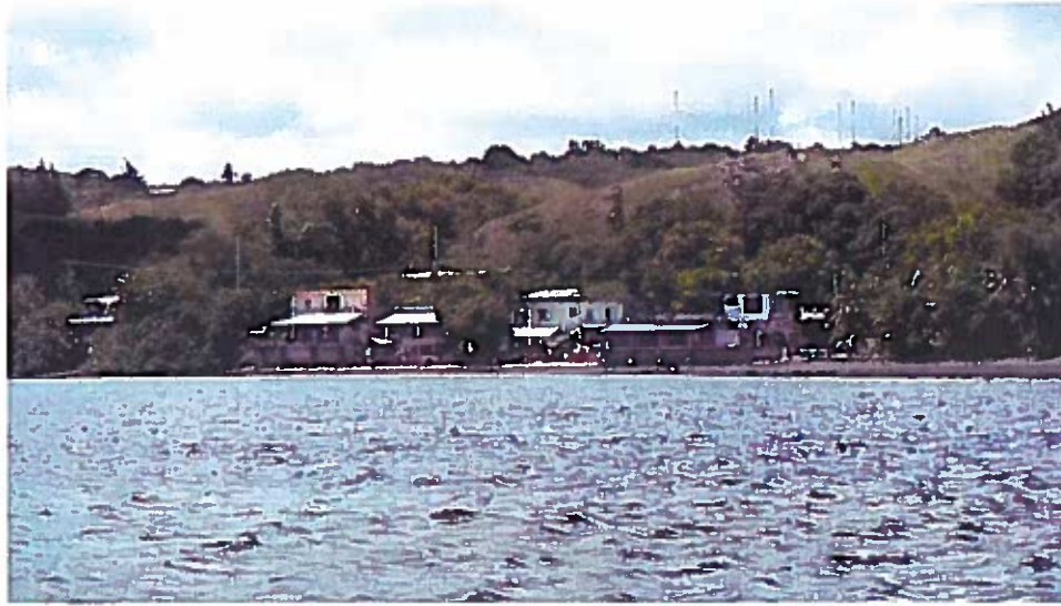
Figure 13. Houses in the town of Merizo bordering Cocos Lagoon.
