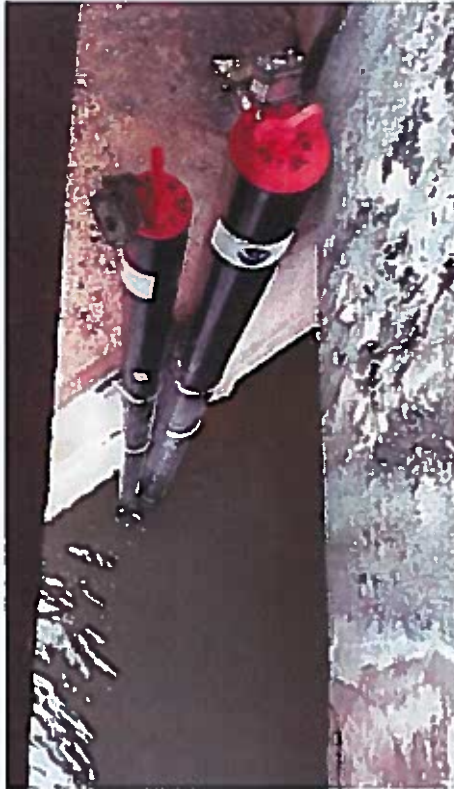
Figure 5. Photograph of turbidity logger (right) and level logger (left) housings attached to the Ajayan River bridge abutment.
